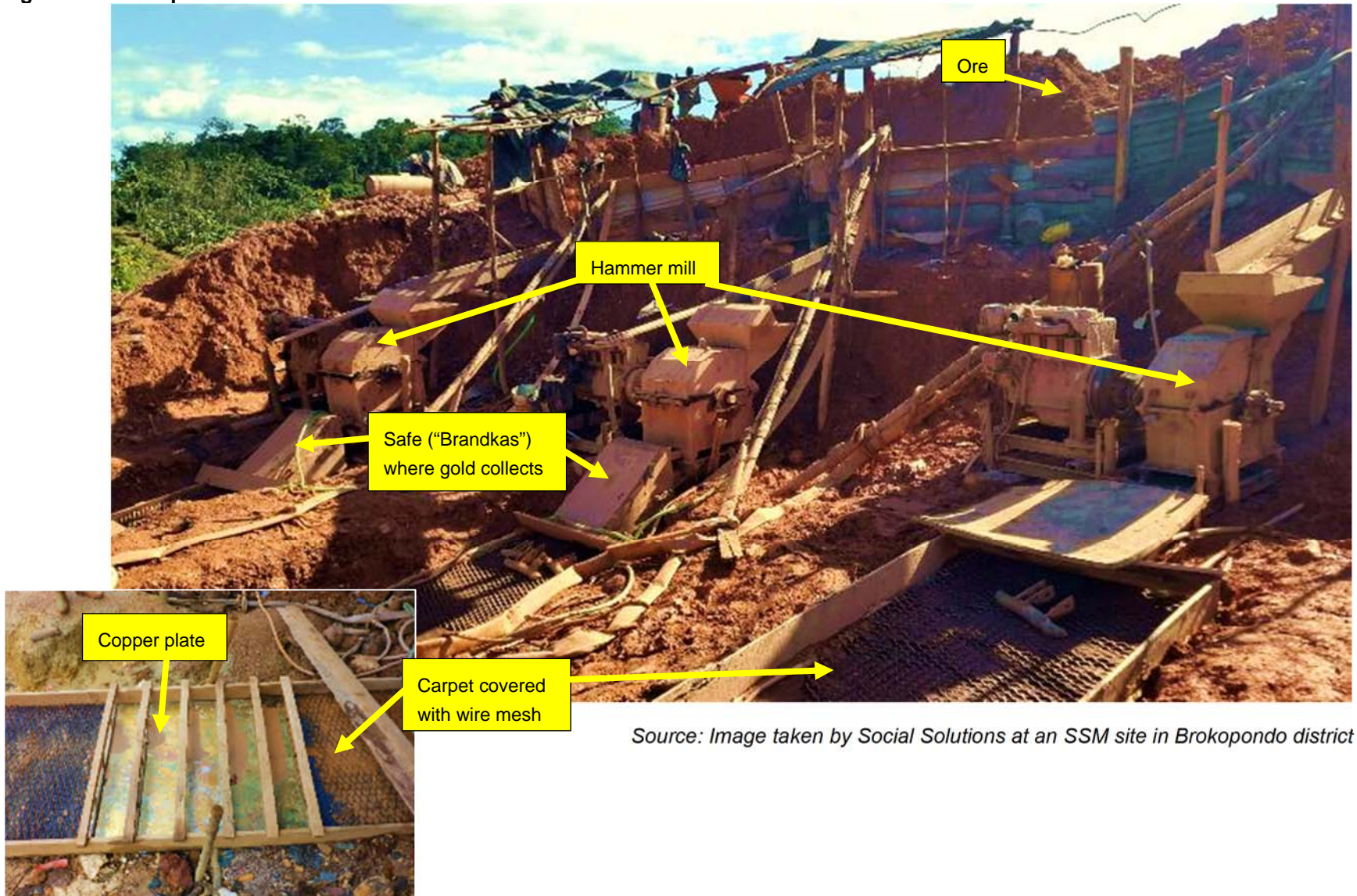
Figure 14. Line-Up of Hammer Mills
