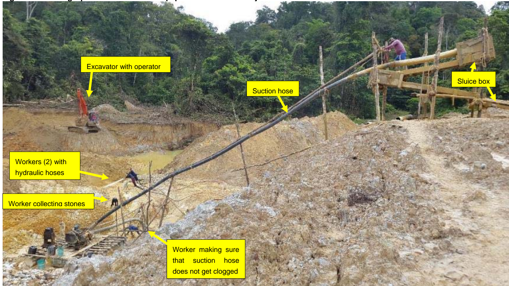
Figure 13. Sluicing Operation of Brazilian Equipment Owner at Sabajo
